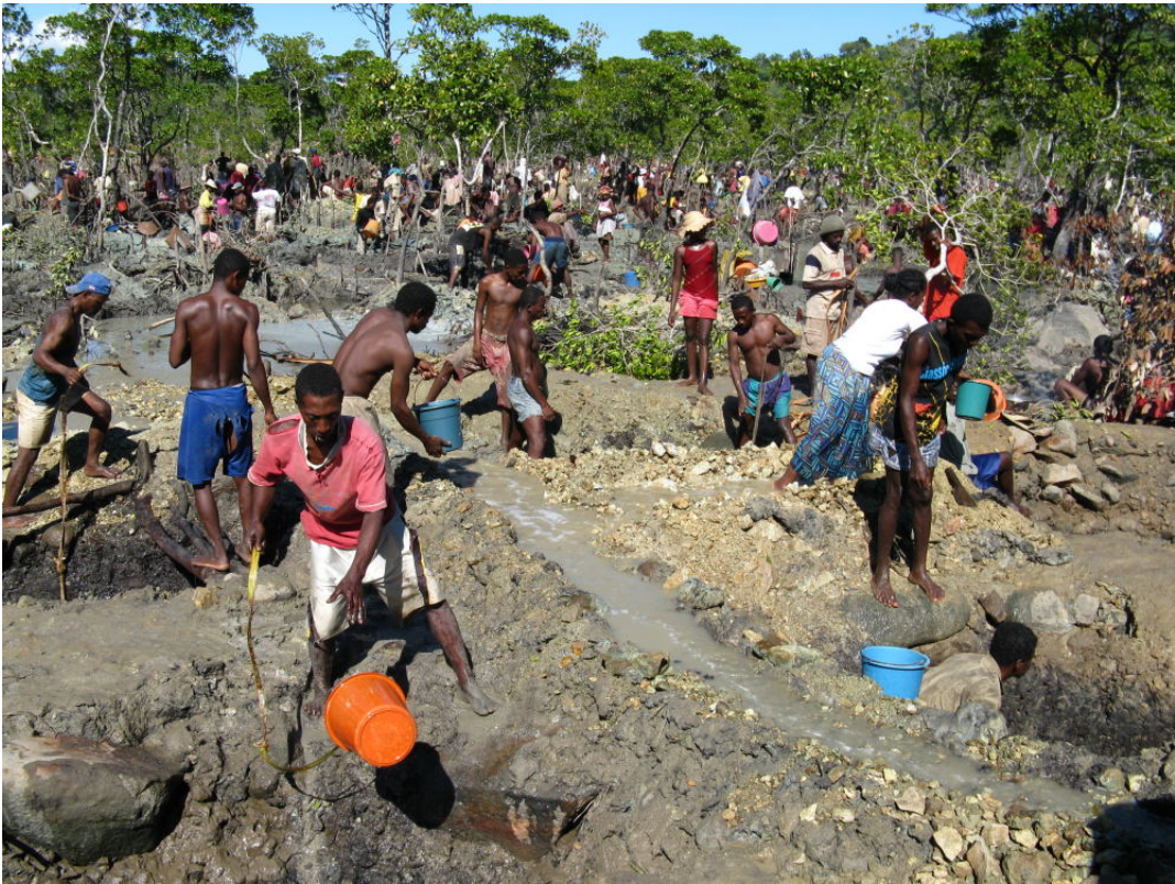
Figure 9. Miners building a drainage canal.
